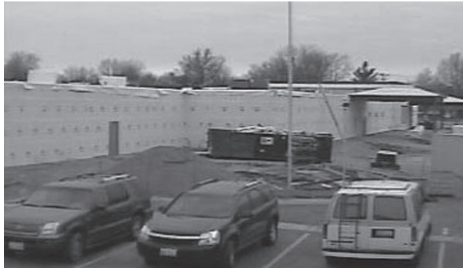
Hamilton Memorial Hospital under renovation
